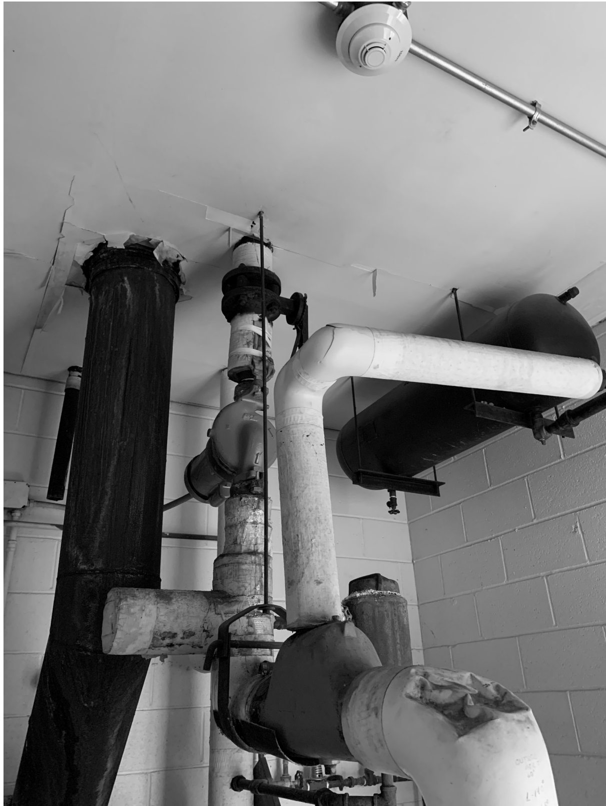
EXISTING BOILER FLUE, PIPING, PUMP, EXPANSION TANK TO BE DISCONNECTED AND REMOVED
