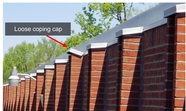
Section F – Loose sheet metal coping cap
