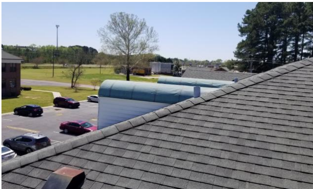
Asphalt / fiberglass shingles and copper topped dormer / louvers
