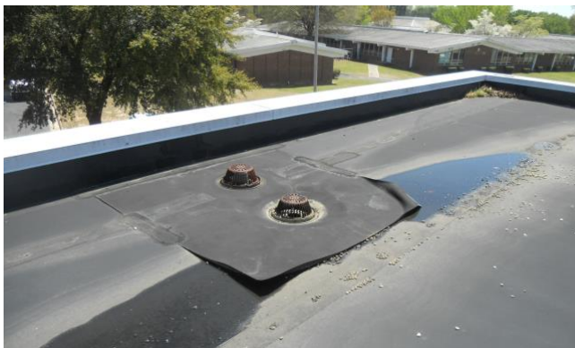
Section H – Ponding water and failed drain target sheet
