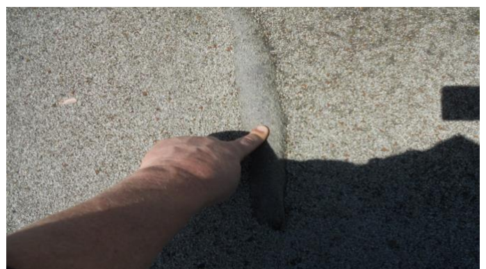
Minor blister in modified bitumen
