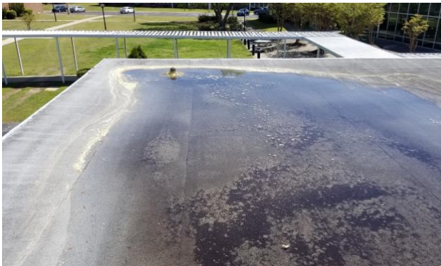
Blocked drain and significant ponding water
