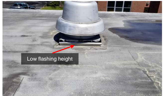
Low flashing height at exhaust fan
