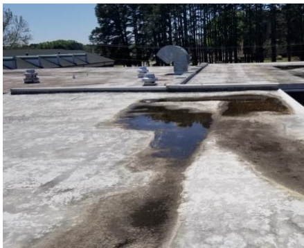
Drainage issues and ponding – Sections E and F
