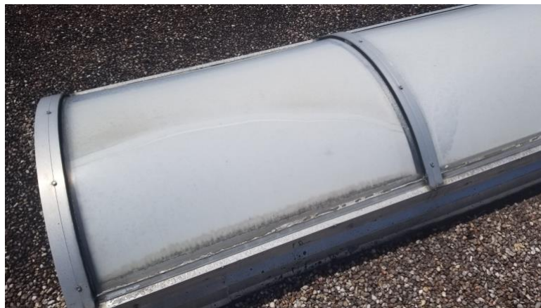
Cracked skylight with water between the domes
