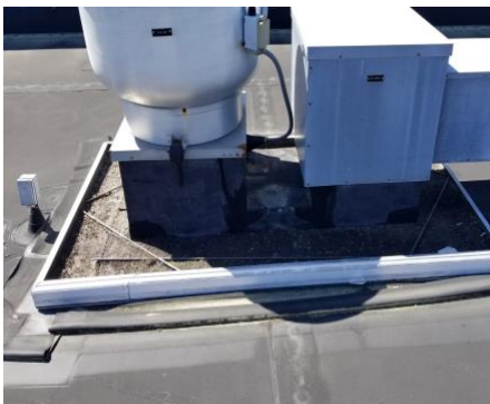
Section B – Grease collector that must be maintained
