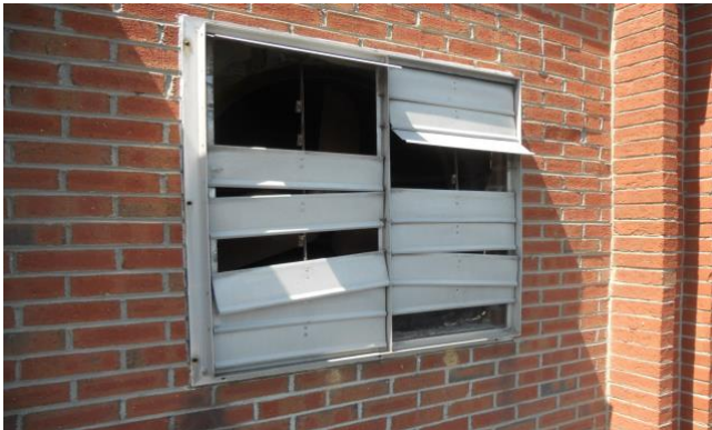
Section H – Louver slats missing can allow water intrusion at roof level
