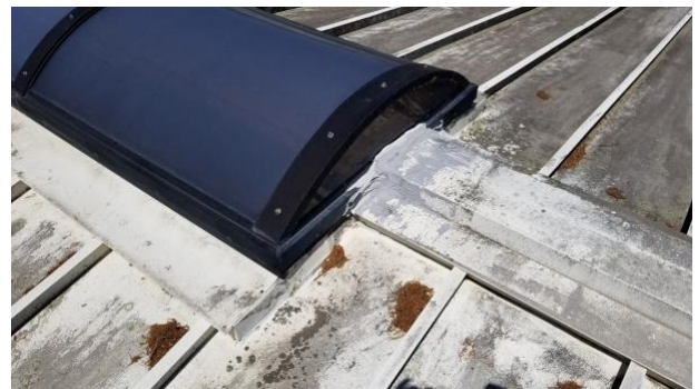
Skylight sealant joint
