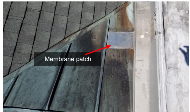
Standing seam metal roof at connector between ILC and Vestal
