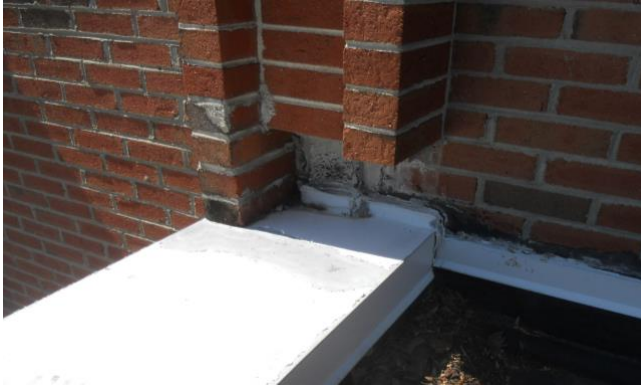
Section H – Poor coping to wall transition.
