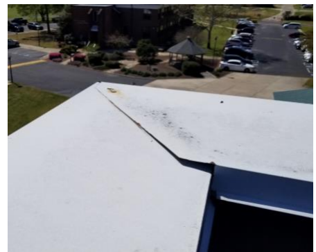
Section C – Open corner coping joint
