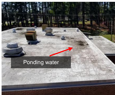
Ponding water and poor coating condition – Sections A & C
