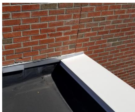
Section B – Counterflashing repair at spalled brick
