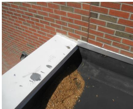
Section B – Debris on roof and peeling coping finish
