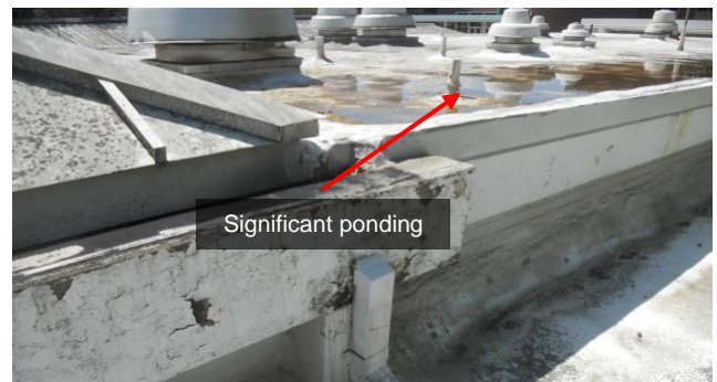
Intersection of low slope roof and steep roof
