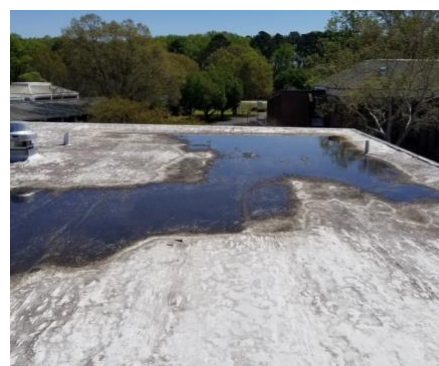
Ponding water on Section F
