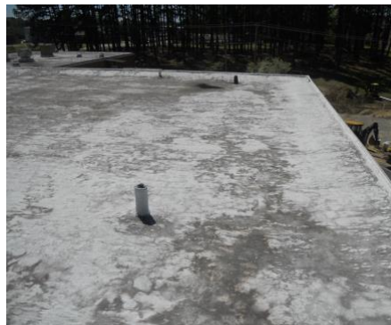
Coating in poor condition – Section E
