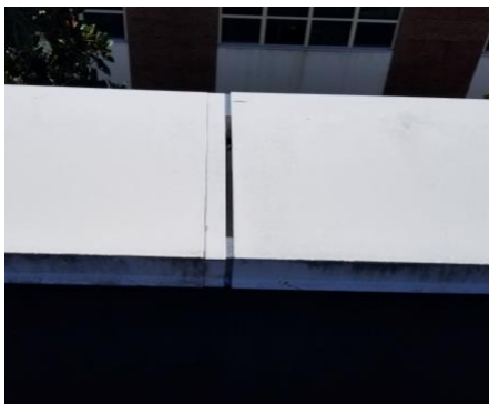
Section A – Open coping joint
