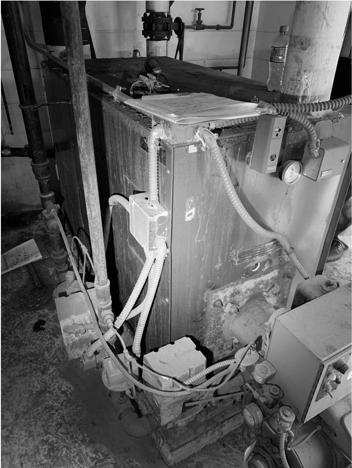
DISCONNECT EXISTING BOILER AND BURNER FROM FUEL SOURCE, ELECTRICAL, AND PIPING CONNECTIONS AND REMOVE. HOUSEKEEPING PAD MAY BE REUSED.
