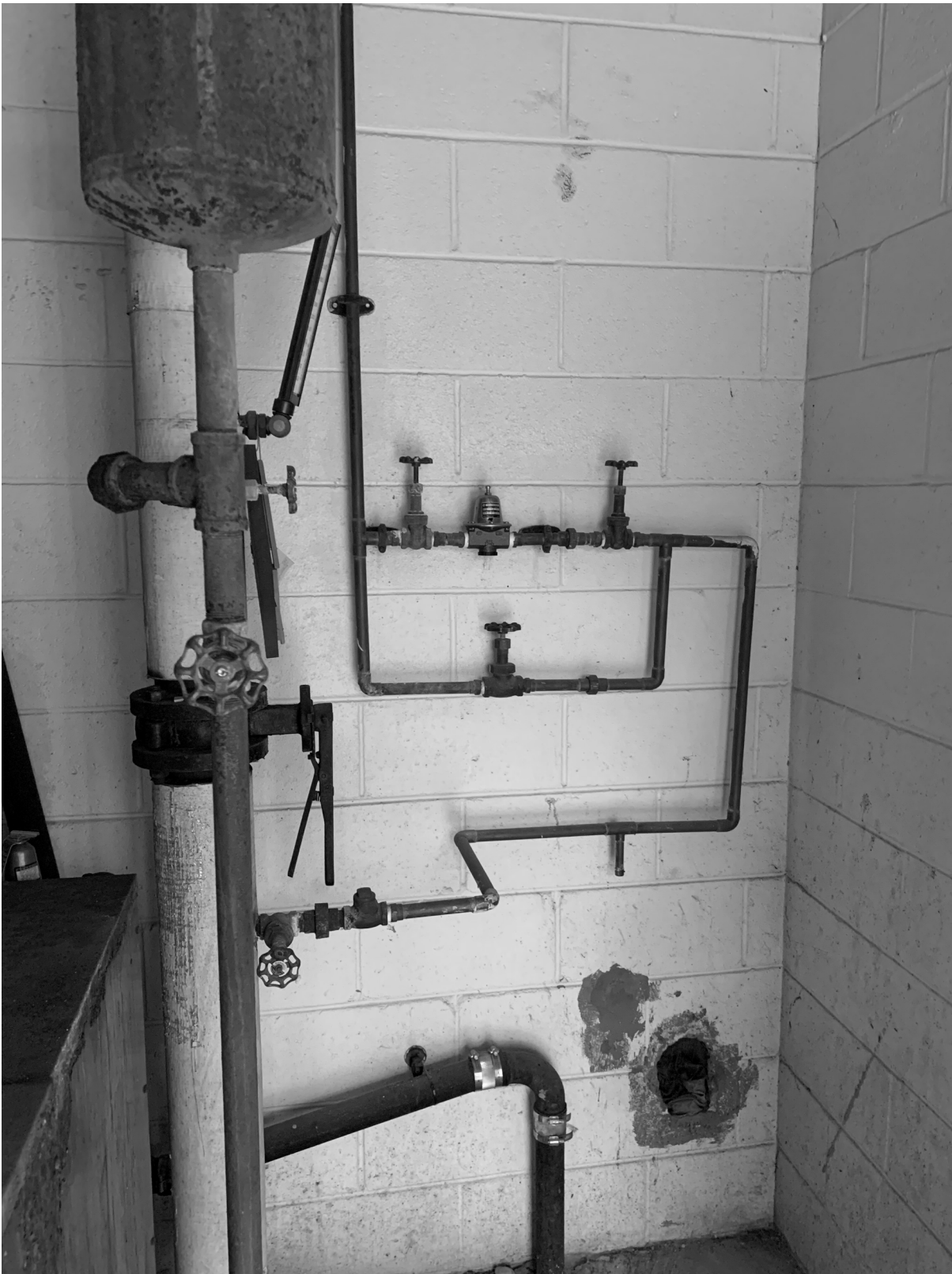
EXISTING DOMESTIC WATER MAKEUP LINE. PROVIDE RPZ AND REPLACE EXISTING PRV. REFER TO DETAIL.
