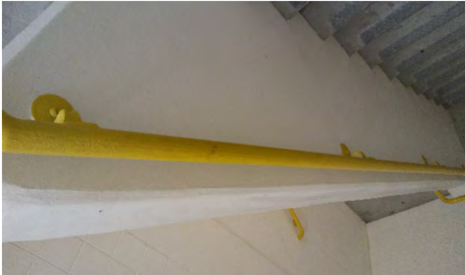
Yellow metal stair railing
