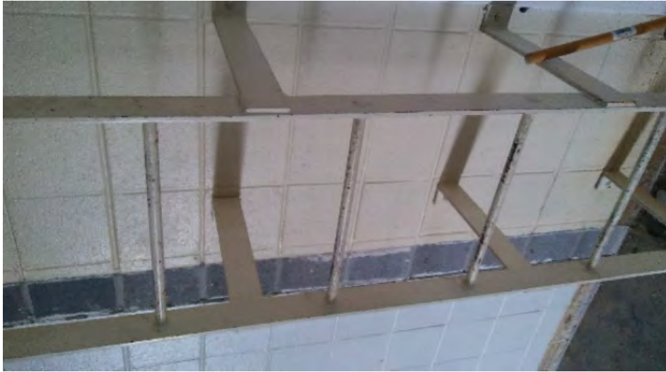
Yellow metal fixed ladder
