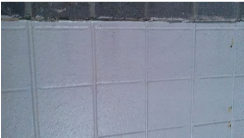
White concrete walls
