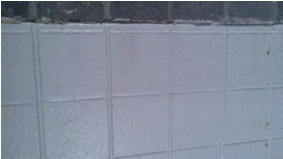
White concrete walls
