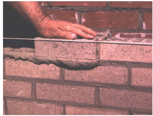
Photo 1 Shoving Brick into Place
